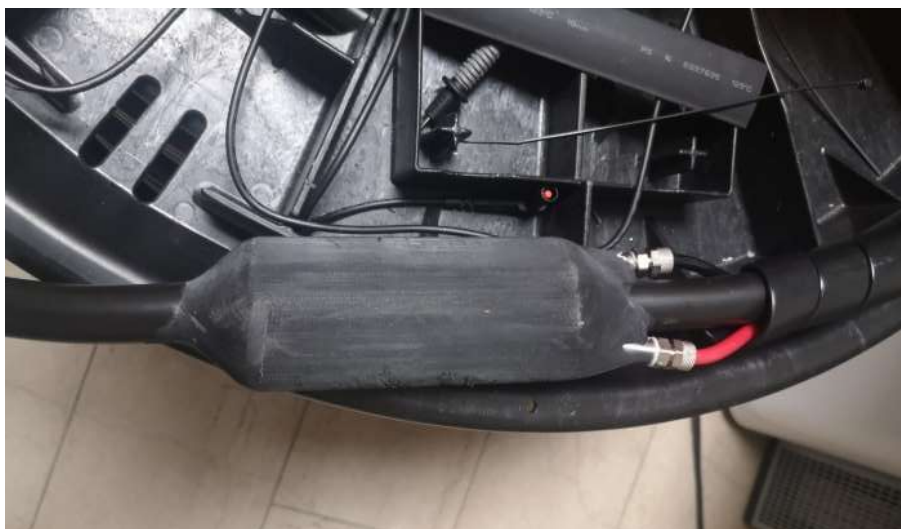
Figure 6: Air split with two air outlets to station 1-4 and 5-8 at about 50cm above the cable split.
